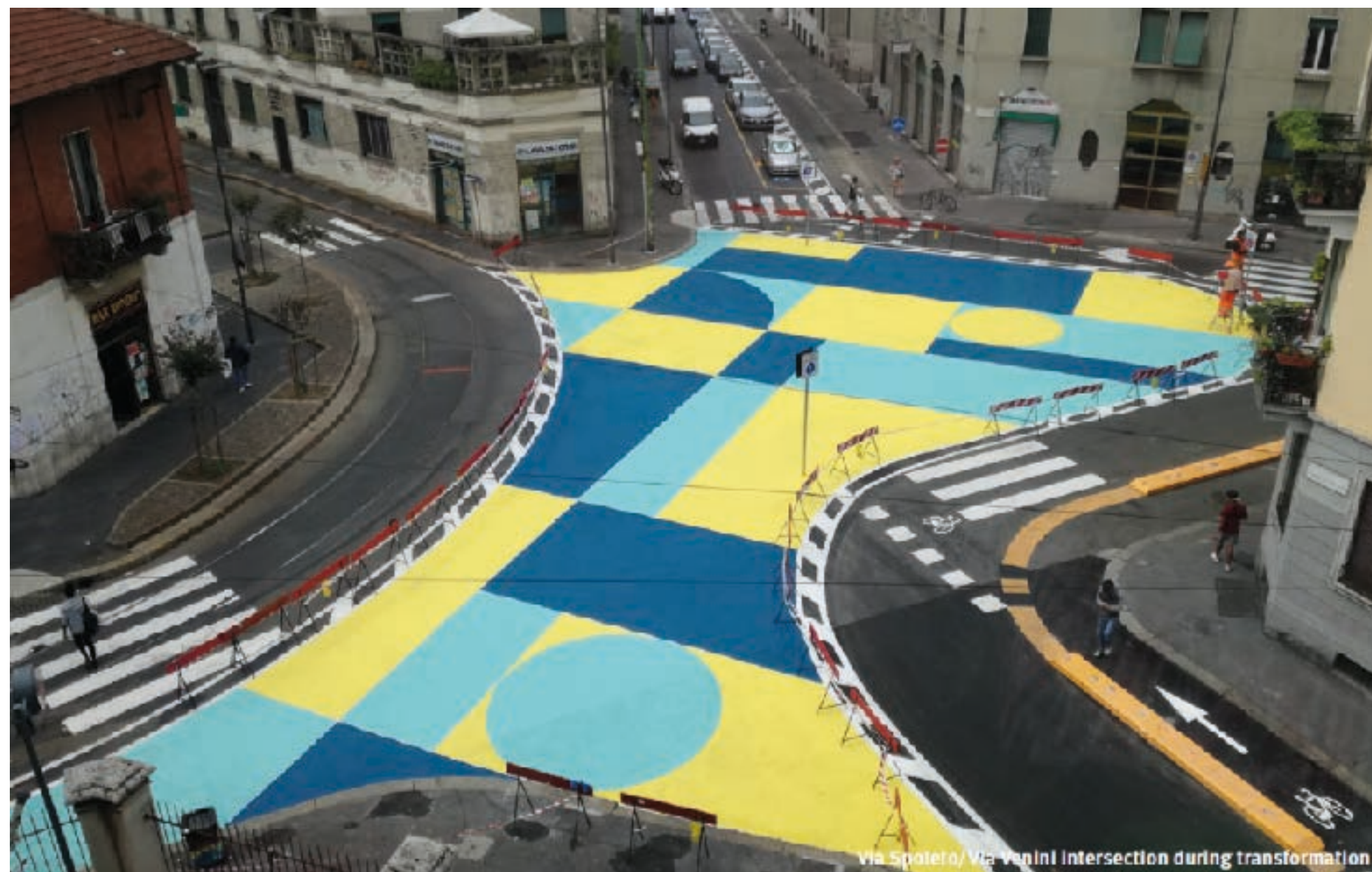
Via Spoleto/Via Venini Intersection during transformation
